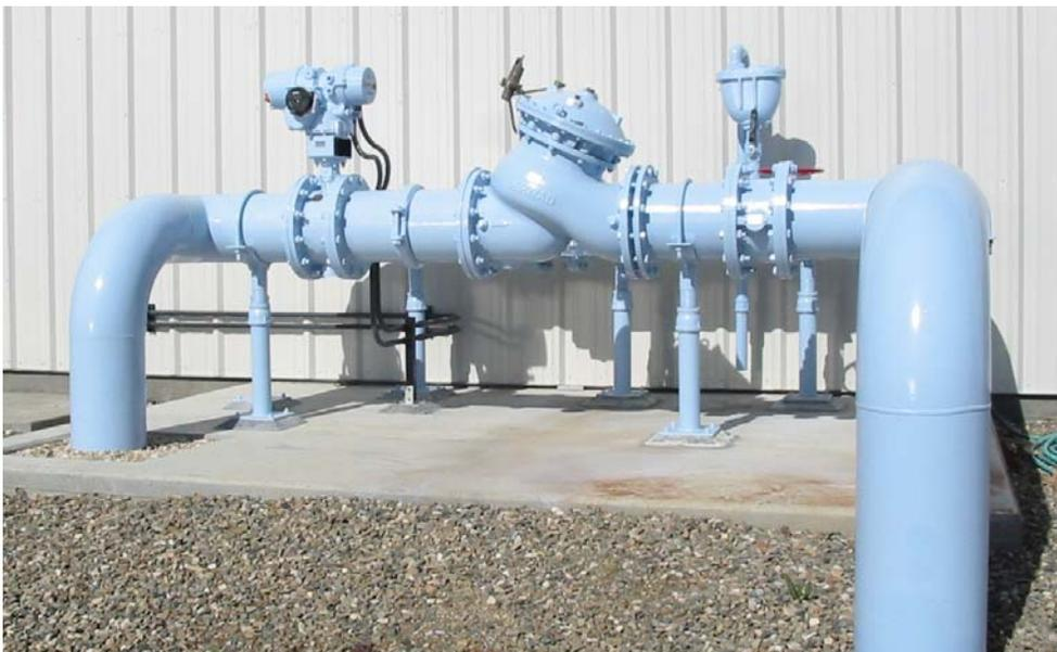
***Air is being drawn into the filtered water through the vacuum valve on the right***
