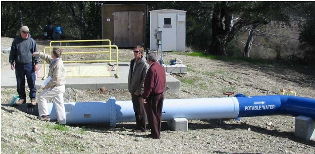
***Ammonia injection could be causing calcium carbonate scaling in the static mixer.***
