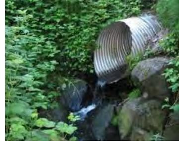
*Point Source Discharge Pipeline*
