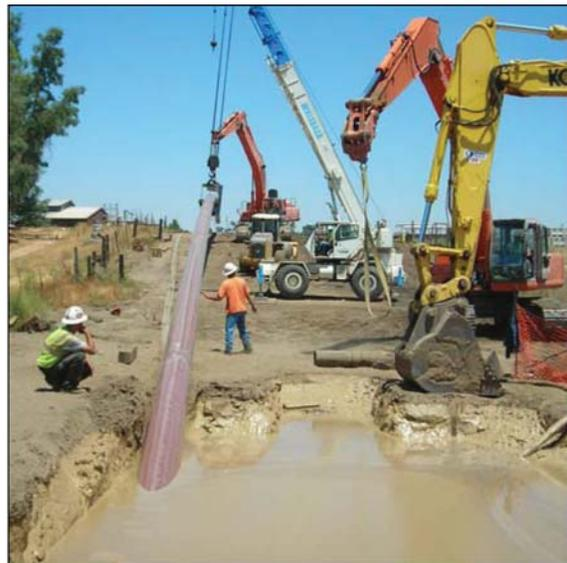
**Figure 3. Atascadero Turnout HDD Pullback**
