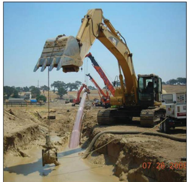
**Figure 4. Paso Robles Turnout HDD Pullback.**
