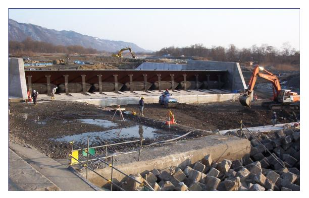
Exhibit A – Typical Installation of Obermeyer Gates
