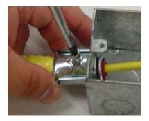
Figure 2 Interlock Armor Bonded. Optical Cable Core Continues
