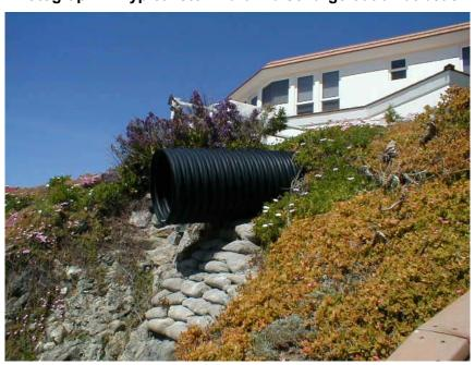
Photograph 3: Caltrans 42-inch culvert outlet near elementary school – Zone 3
