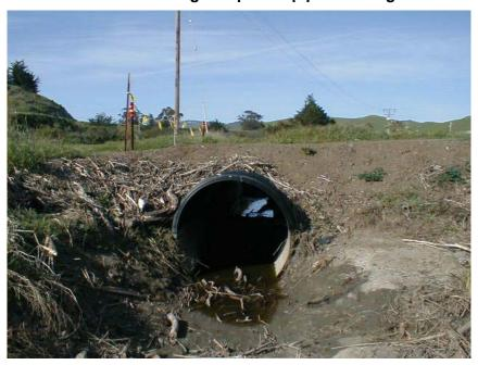
Photograph 8: 30-inch reinforced concrete pipe culvert at Park Avenue upstream of Third Street drain
