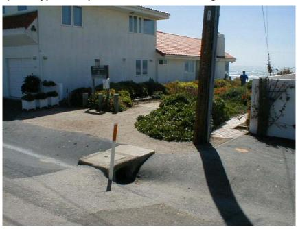
Photograph 2: Typical storm drain discharge outfall at beach
