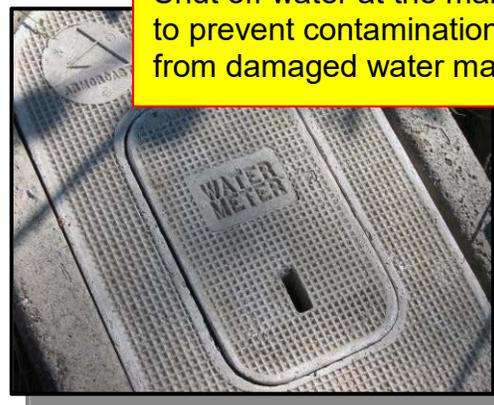
Shut off water at the main to prevent contamination from damaged water main
