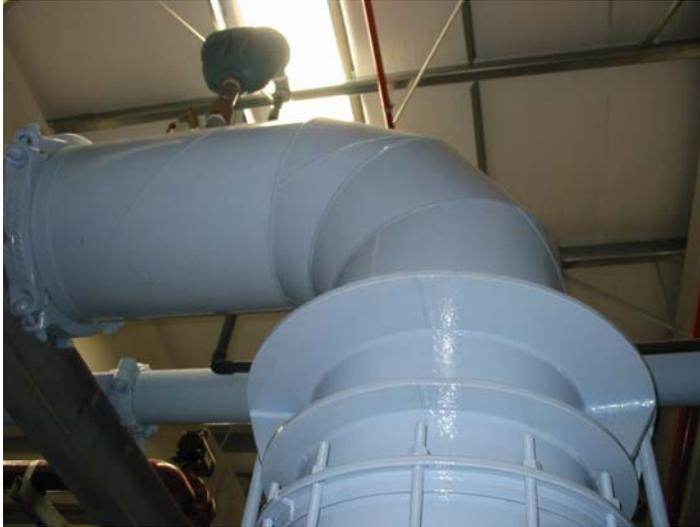
***Air/vacuum valve on MF filtrate piping***
