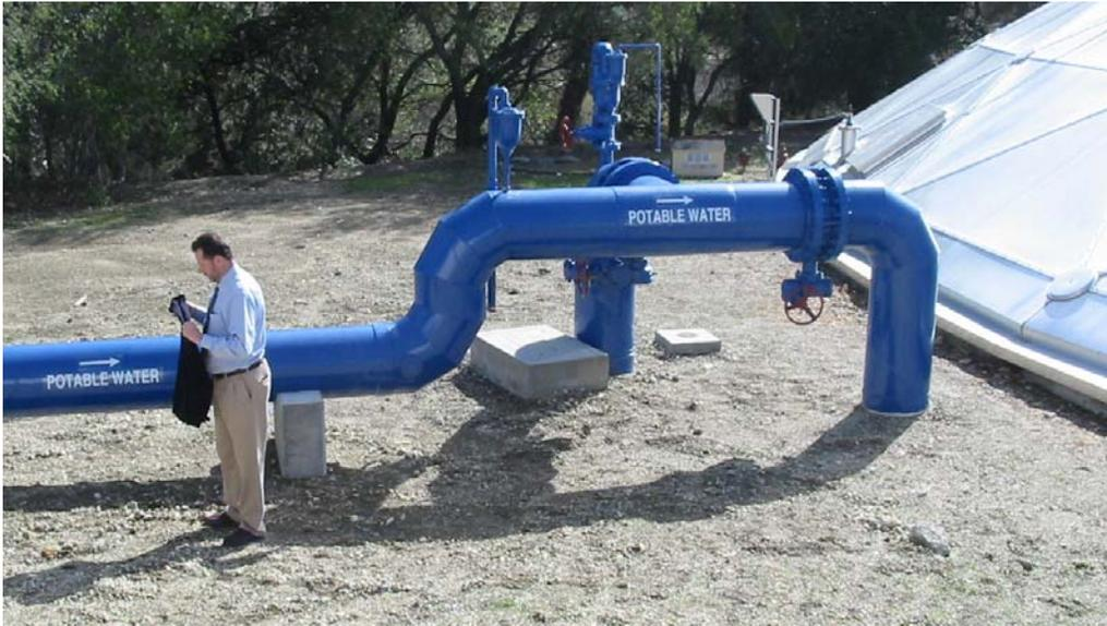
***Air is being drawn into the filtered water through the vacuum valve on the left***
