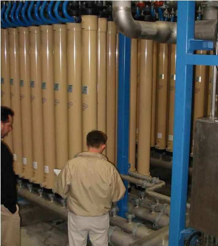
***Lopez WTP MF skid. Notice connections for 6 additional elements per skid at lower right.***
