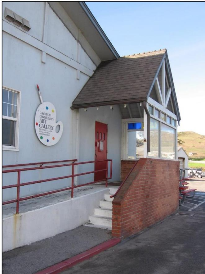
**Figure 43.** Modern signage, access ramp, stairs, railings, door, and glass-enclosed portico associated with Cayucos Community Art Gallery portion of Cass Warehouse building. The doorway itself is probably original to the warehouse building (compare with Figure 29, above).
