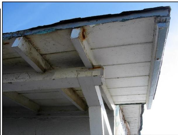
**Figures 47 and 48.** Details of shed-roof extension of roof line on west elevation, sheltering row of windows and doorway. These are not original historic-period features of the Cass Warehouse (compare with Figure 26, above).
