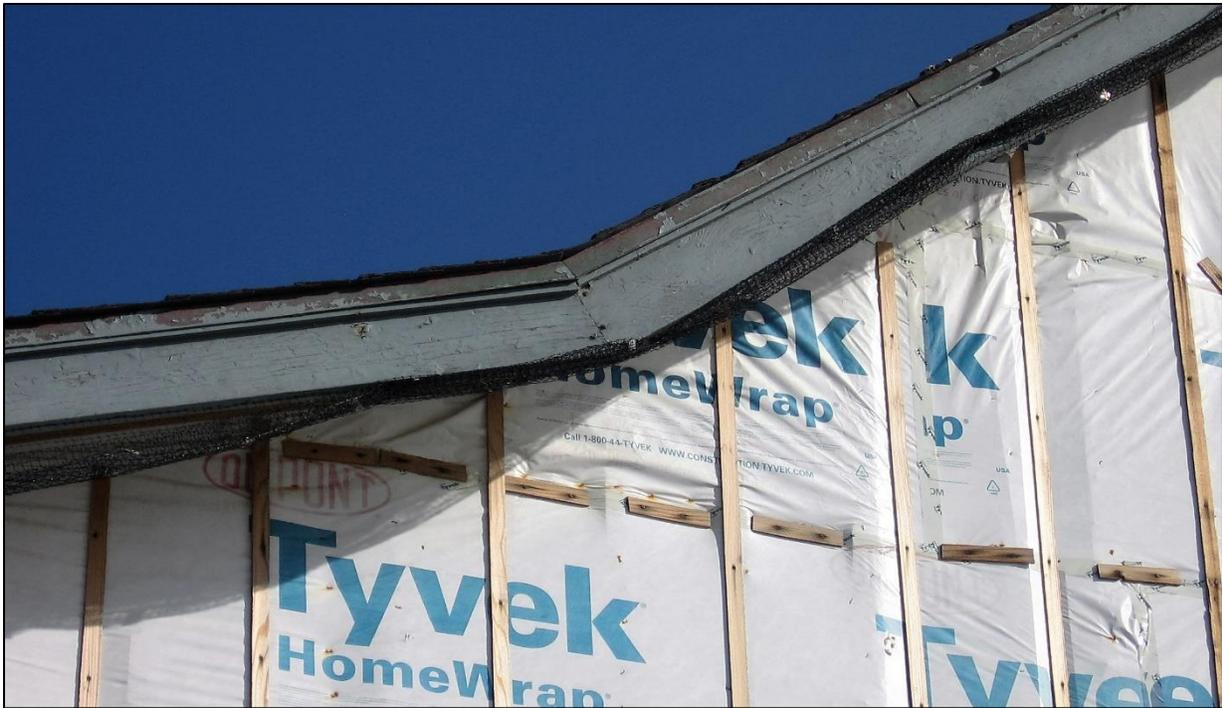
**Figure 45.** Original historic-period roof plane articulation on rear elevation. The fascia is probably original, although the flashing was probably added with the new roofing material (Compare with Figure 23, above).
