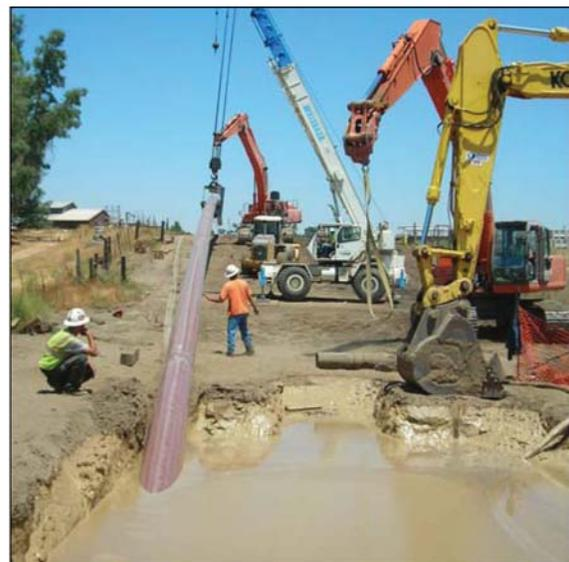
**Figure 3. Atascadero Turnout HDD Pullback**
