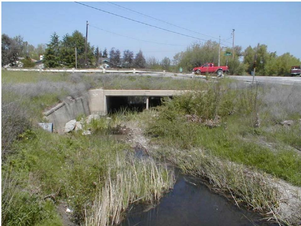
**Photograph 3: Excessive Vegetal Growth downstream of I Street Culvert Crossing**
