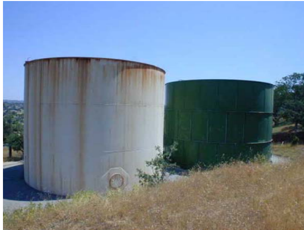
Figure 4-3: Existing Storage Tanks Reservoir 01 (left) and Reservoir 02 (right)
