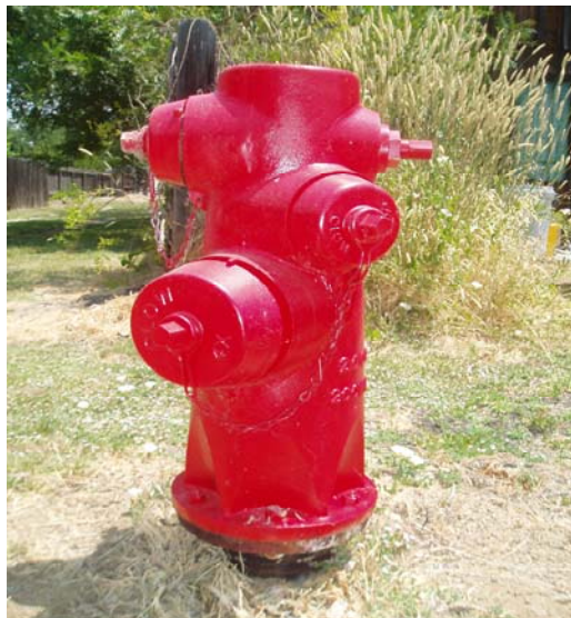
Figure 4-4: One of the 17 New Hydrants installed
