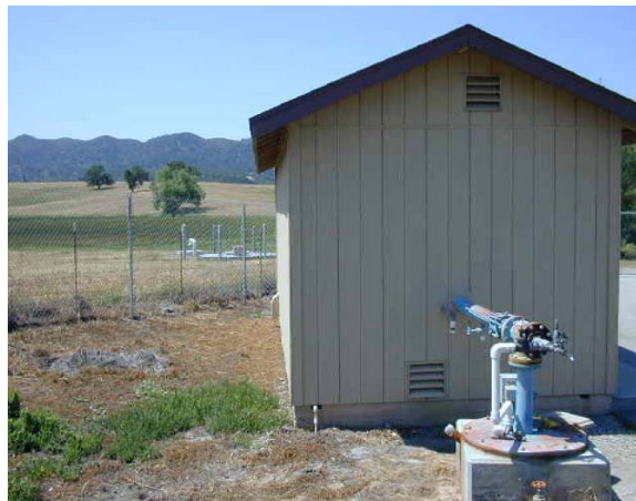
Figure 4-1: Well 3 Pump House
