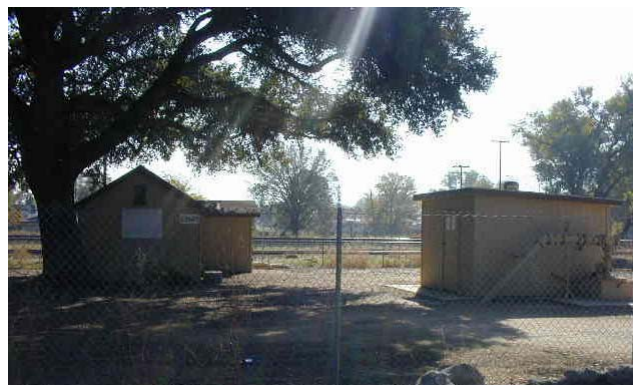
Figure 4-2: Well 4 Pump House (left) and Wells 1 & 2 Pump House (right)
