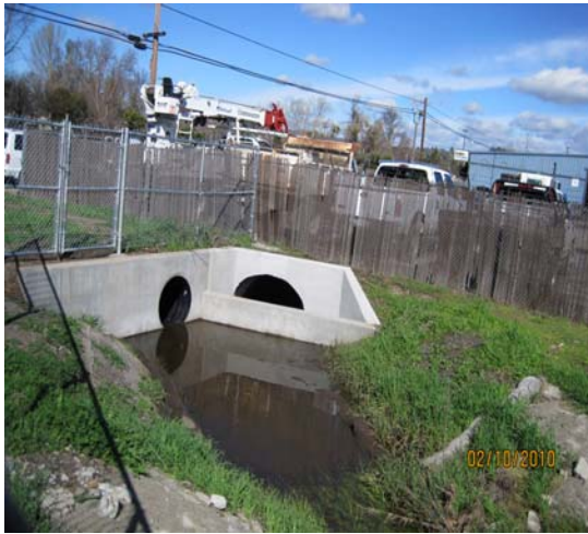
Inlet at Highway 58
