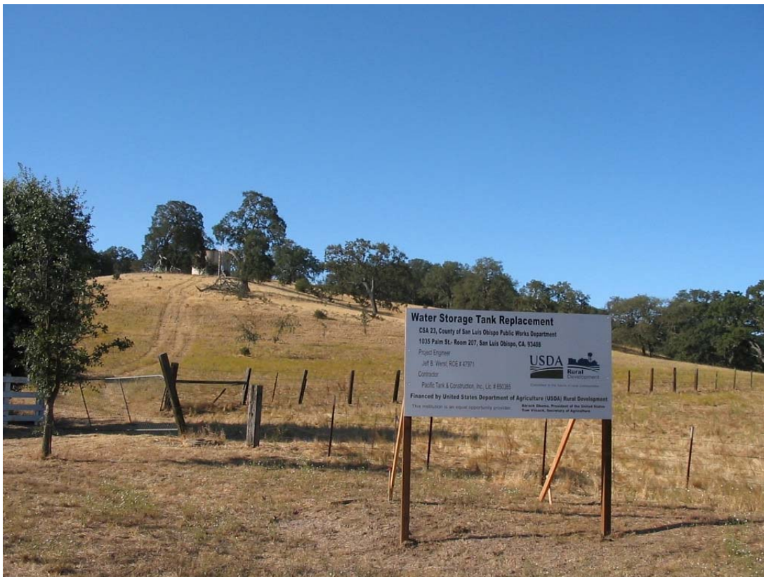
Figure 7-1: Site of the new Water Storage Tank and Access Road (with the existing Reservoir 01 visible at the top of the hill)
