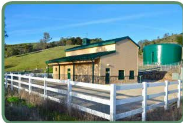
Rocky Canyon Pump Station and Tank
