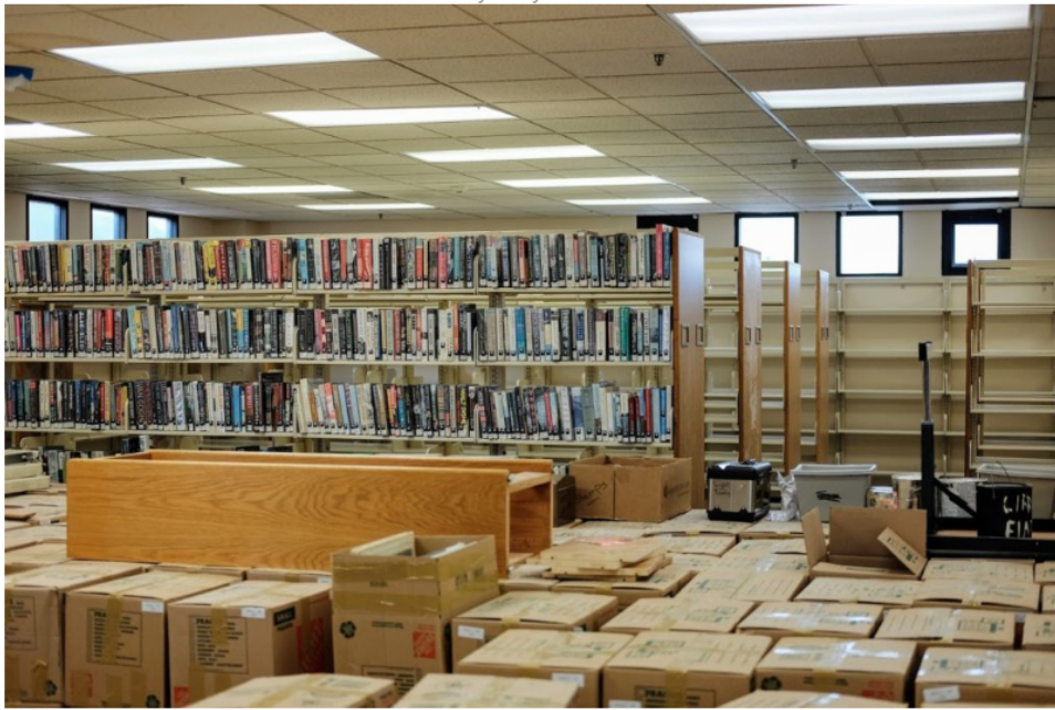
County library renovation
