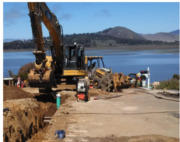
Construction of Los Osos water pipelines.
