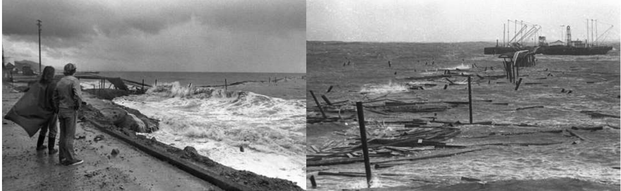
Figure 5- 36 Union Oil Pier in Avila Beach Collapses Following Severe 1983 Storm
