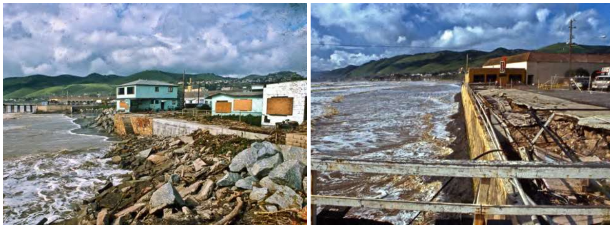
Figure 5-32 Coastal Storm Damage at Pismo Beach, 1982/83 El Niño
