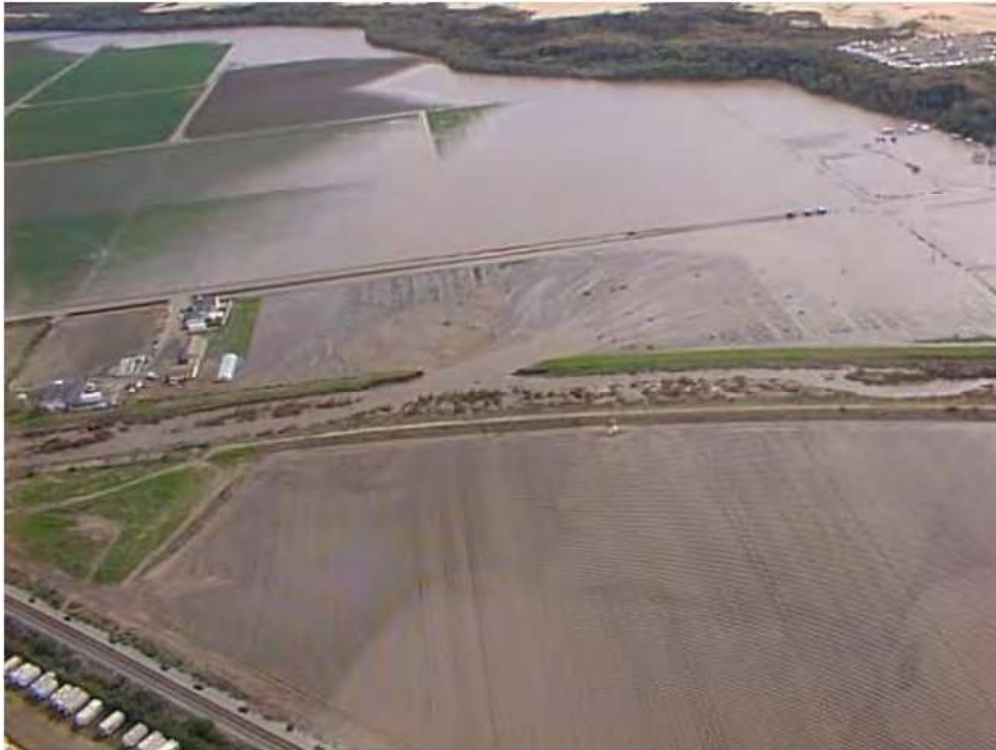
Figure 5-69 Arroyo Grande Levee Failure Event, March 2001 (Looking South)
