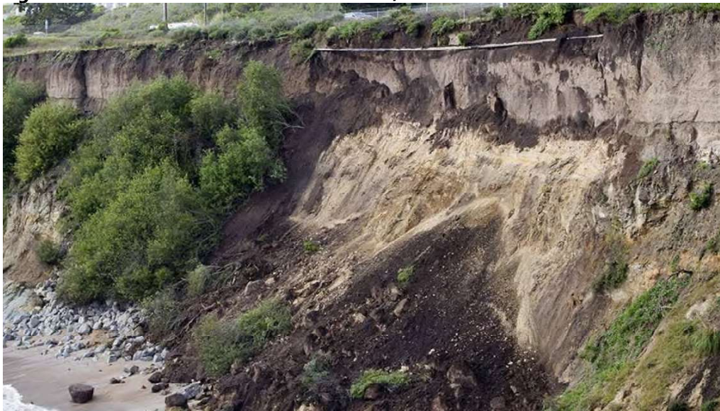
An approximate 100-foot section of cliff collapsed in Pismo Beach due to erosion of the bluff following winter storms in March 2011, demonstrating the severe impacts of coastal hazards on weak bluff sediments. Source: San Luis Obispo Tribune 2011
