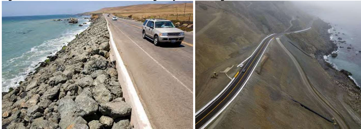
Figure 5-38 Vulnerable Portions of Highway 1 and Realignment near Piedras Blancas
