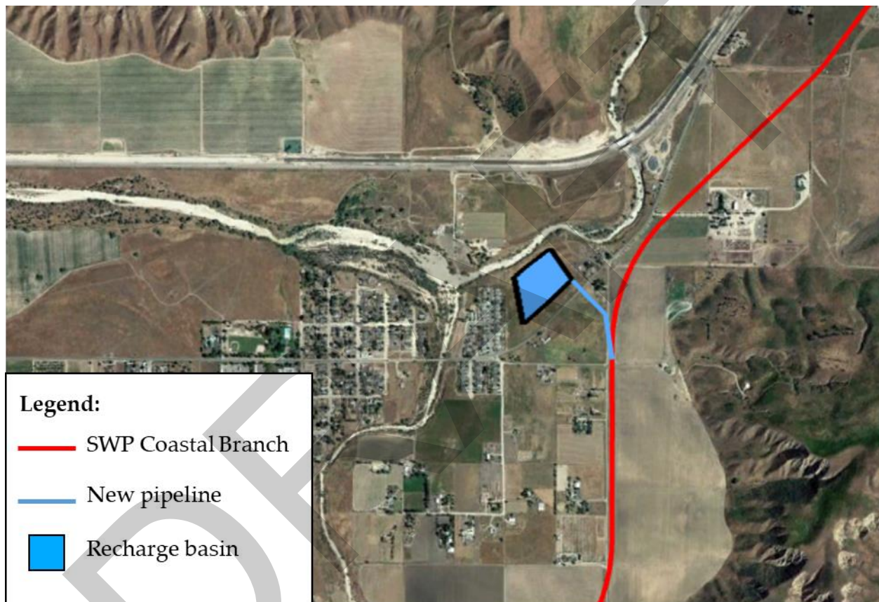
Figure 5. SWP to recharge basin in Shandon
