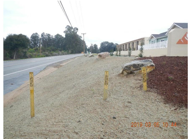
Hydroseed application to cover soil
