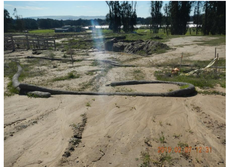
Sediment Control (Straw Wattles)
