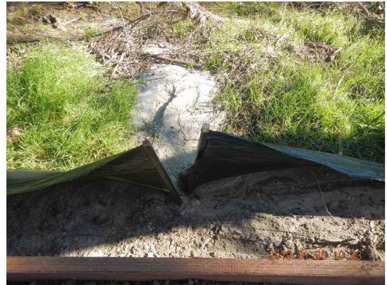
Sediment Control perimeter protection (Silt Fence)
