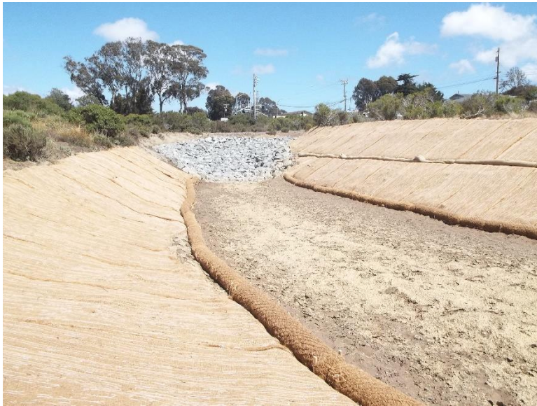
Erosion Control blankets to cover soil
