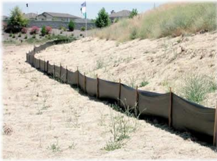
Sediment Control perimeter protection (Silt Fence)
