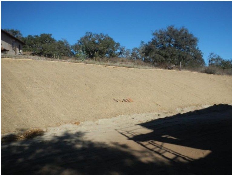
Erosion Control blankets to cover soil
