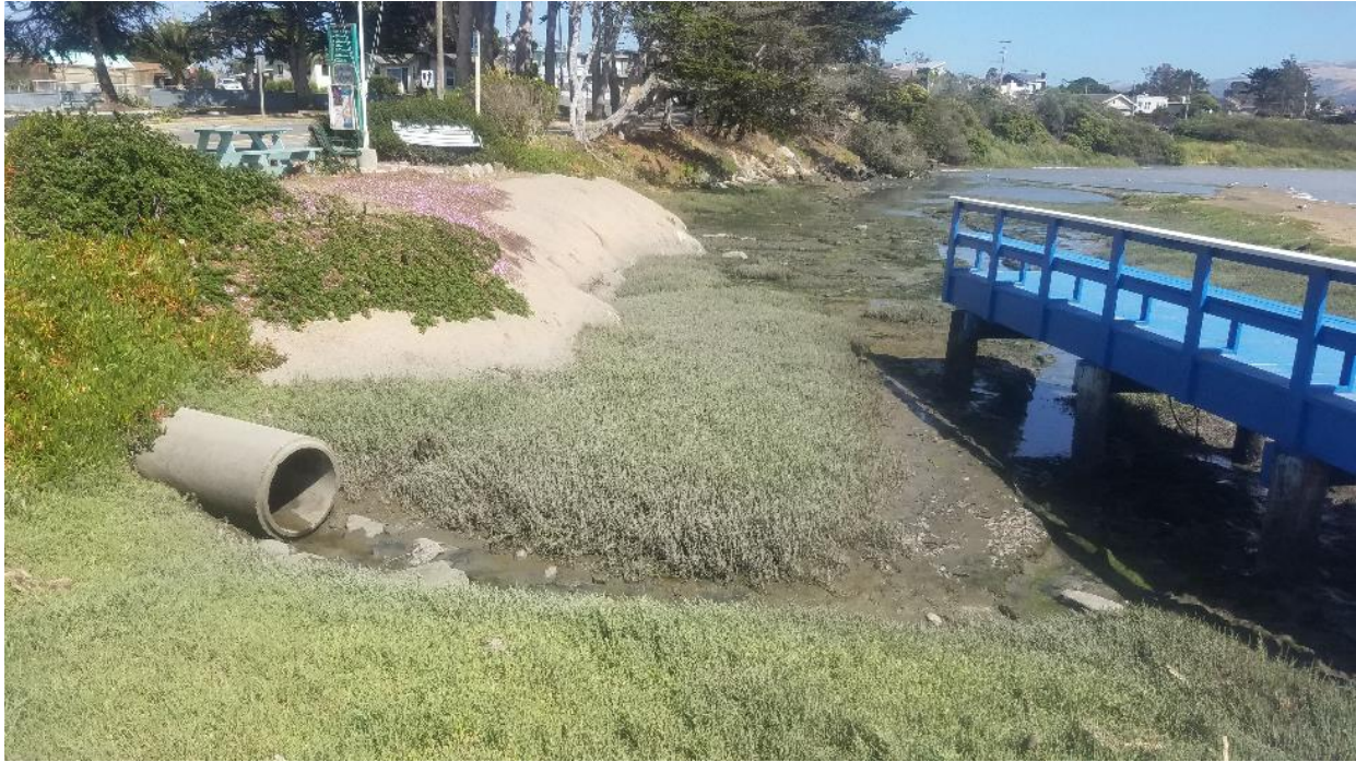
Figure 11. One of the two stormwater outfalls into Morro Bay
