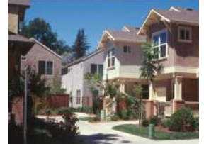
Figure 2-6: Multi-family residential development resembling single-family residential characteristics.
