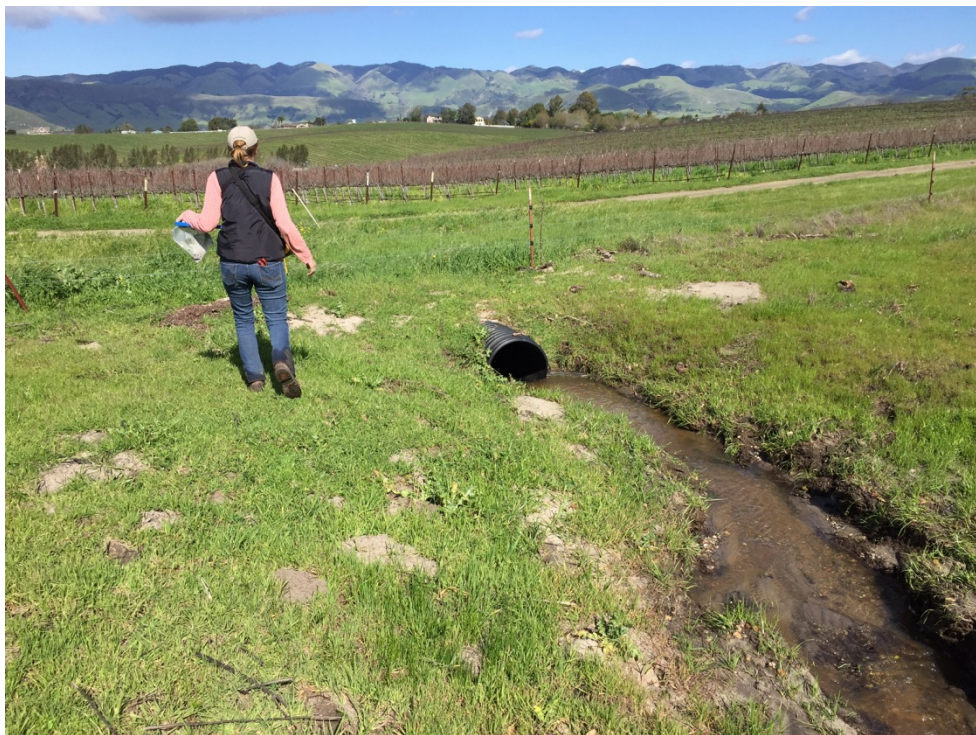
Photo 4: View northwest of the southeastern drainage where it enters a culvert running under the vineyard to the north. This drainage flows into the tributary to Davenport Creek.
