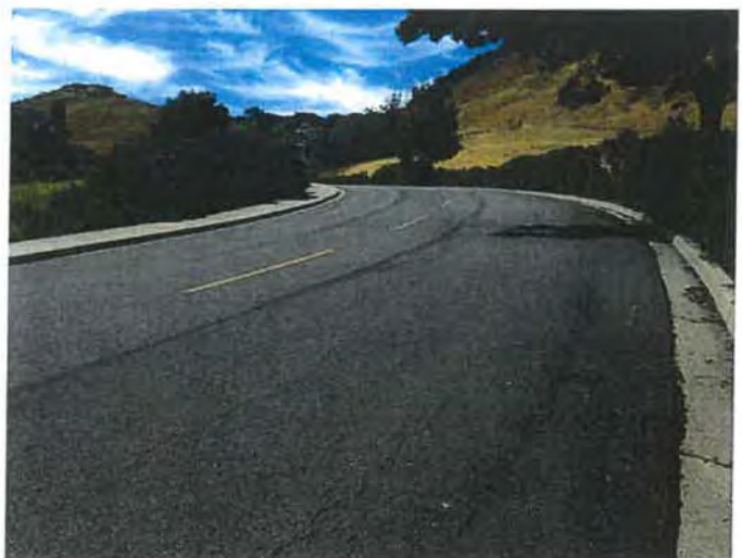
SIGHT DISTANCE TO WEST
