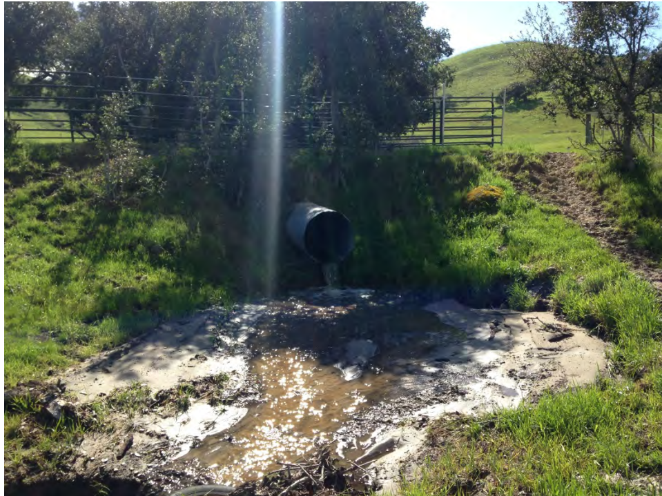
Photo 5: View southwest of the southeastern drainage near the proposed crossing.
