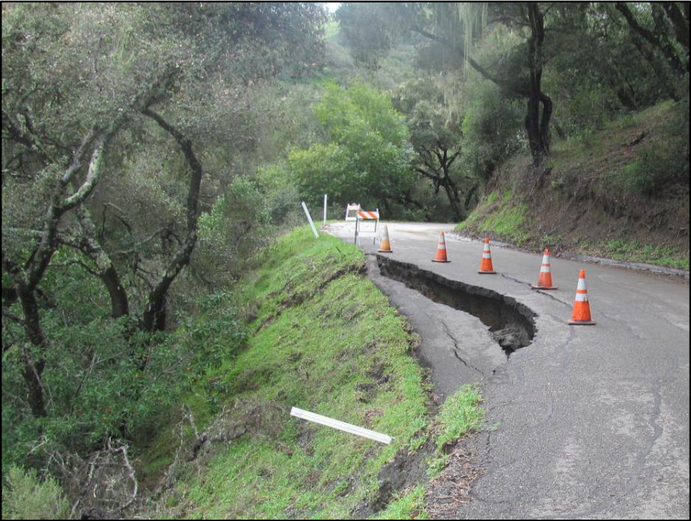
Photo 2. Prefumo Canyon Road MP 3.5
