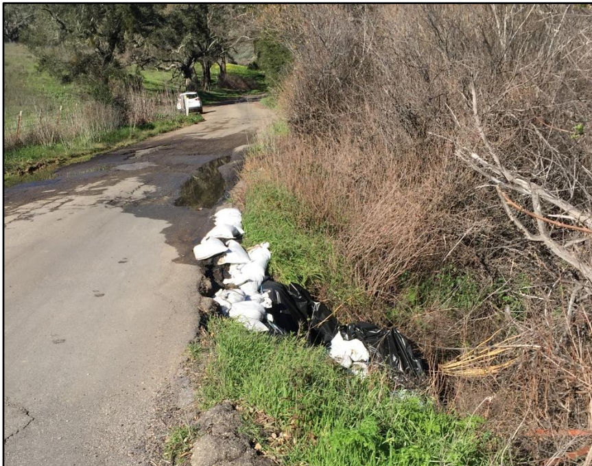
Photo 4. Suey Creek Road MP 1.75
