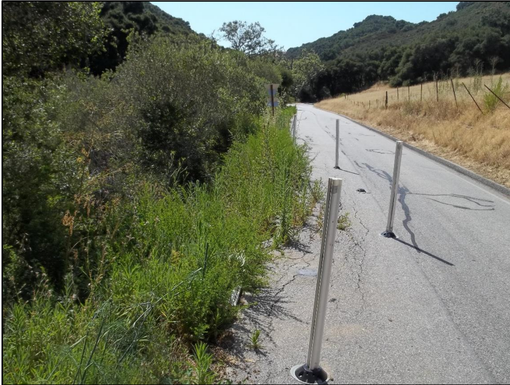
Photo 3. Prefumo Canyon Road MP 3.9
