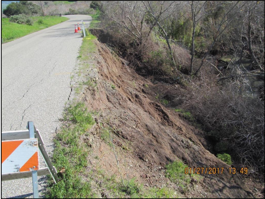
Photo 7. Toro Creek Road MP 1.9
