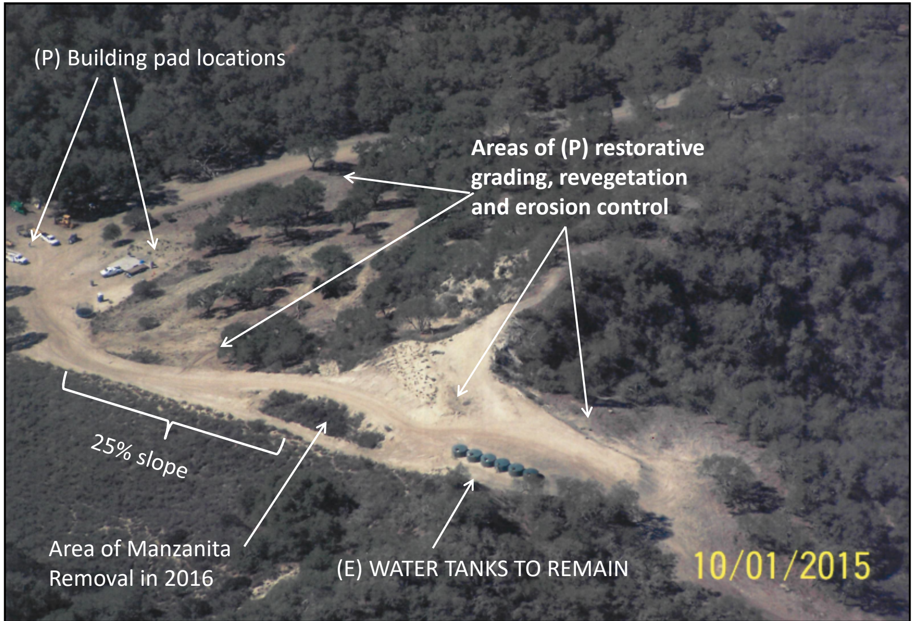
Aerial view of grading remediation area in SW corner of property Viewed from south towards NW
