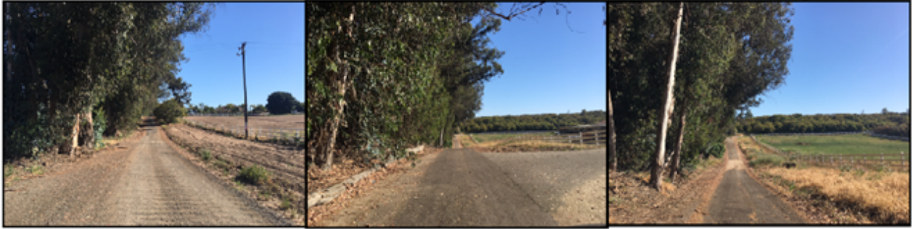
Figure 4 - Three Sections of Albert Way to be Improved (looking north)
