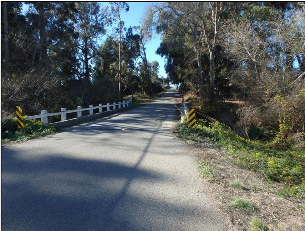
Photo 4: Toro Creek Road Bridge over Toro Creek. Work will occur on both abutments and the stream will be diverted if water is present.
