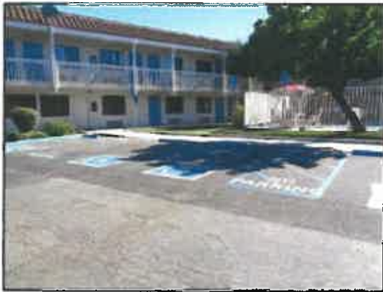
Parking area and swimming pool
