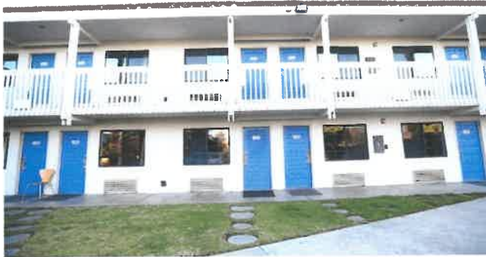
Picture 1: Picture of the east elevation of the Project site. These former guest rooms were turned into office space for the operation of the emergency shelter.
