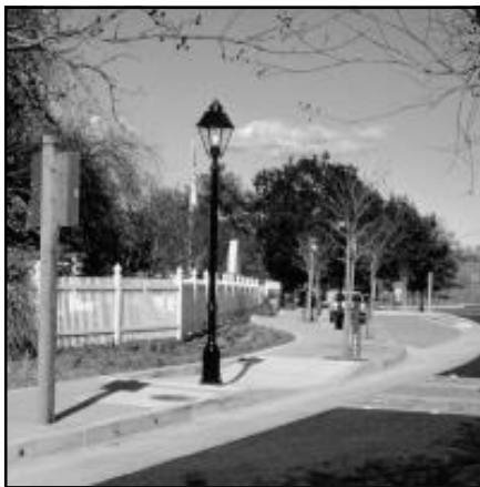
Village Lighting Example
