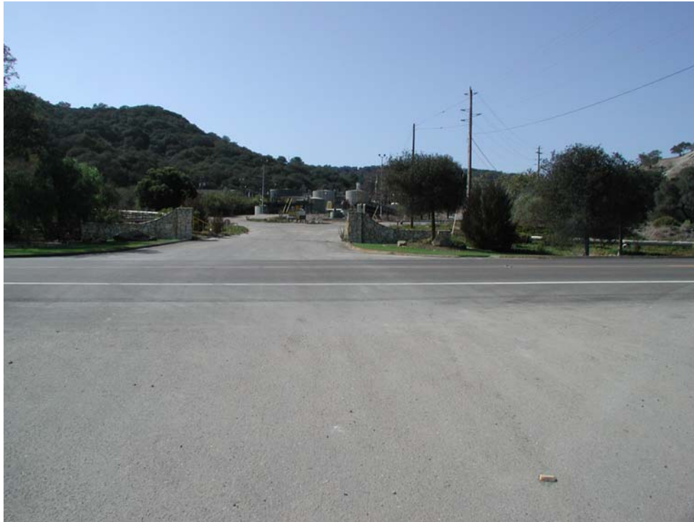
KVA -5 View of Existing Facilities from Price Canyon Road.
