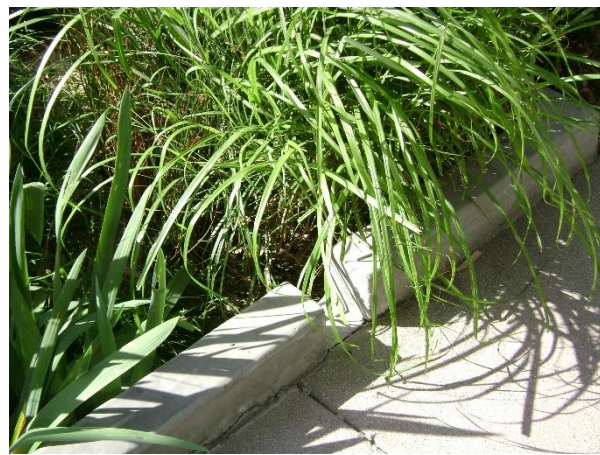
Examples of parkway/LID and curb cuts applications allowing for water infiltration.
