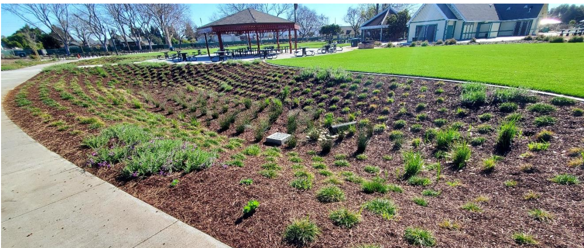
Example of stormwater basin.
