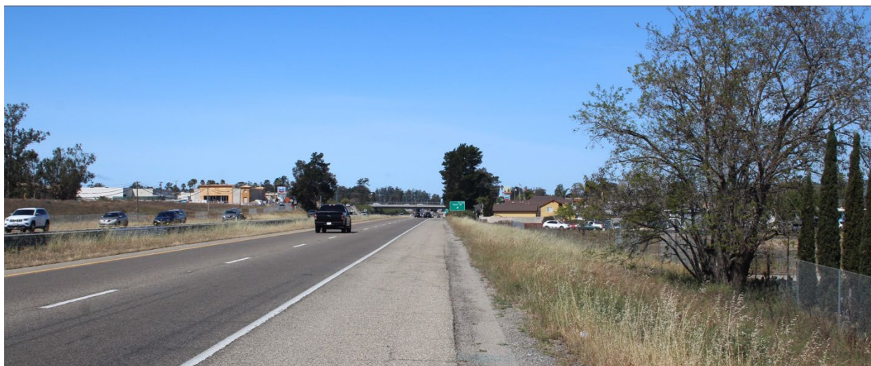
Figure 4.1-13. View along northbound US 101 approaching Tefft Street.
