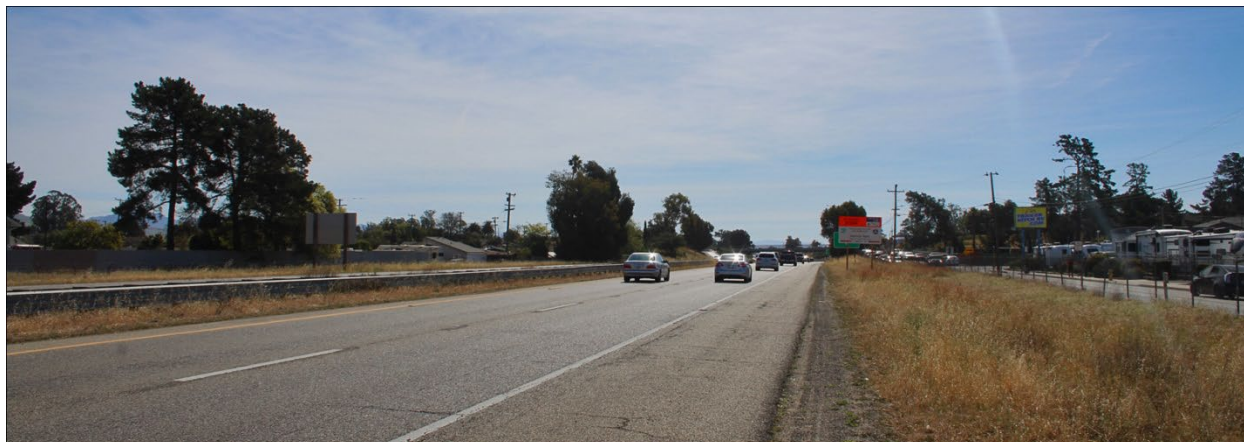
Figure 4.1-12. View along southbound US 101 approaching Tefft Street.
