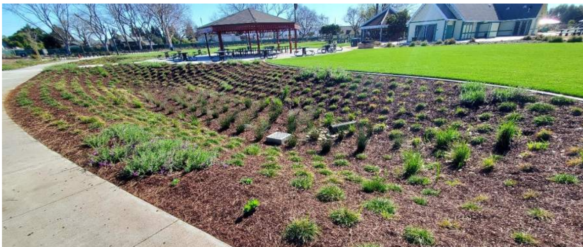
Example of stormwater basin.
