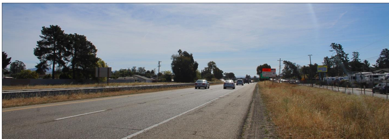
Figure 4.1-12. View along southbound US 101 approaching Tefft Street.
