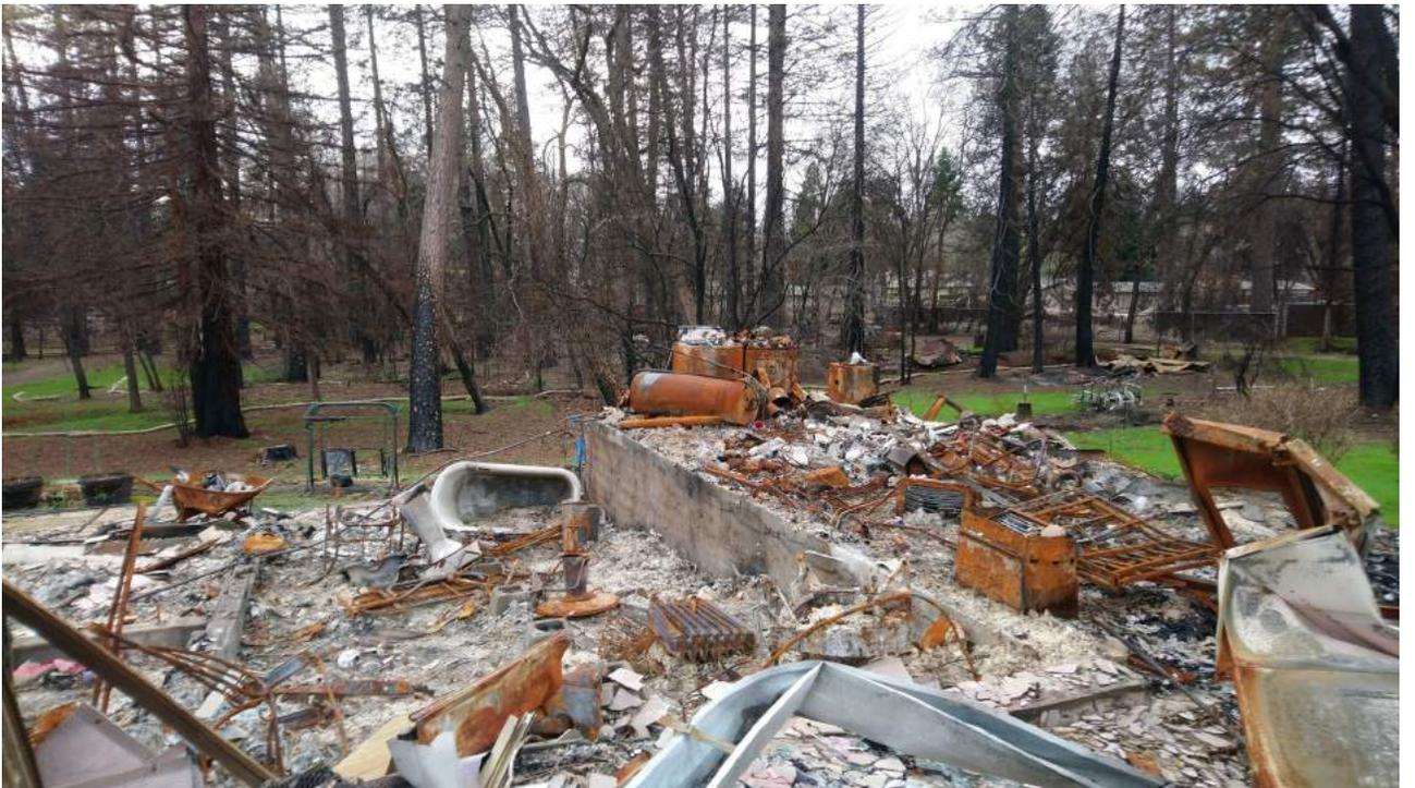
You can see the stucco plaster, which has not burned (after all, it is cement), while all the wooden parts of the house (OSB, 2x4 boards) have burned down completely.
