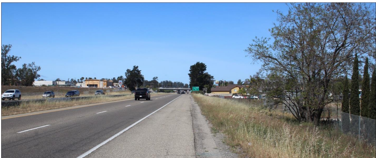
Figure 4.1-13. View along northbound US 101 approaching Tefft Street.
