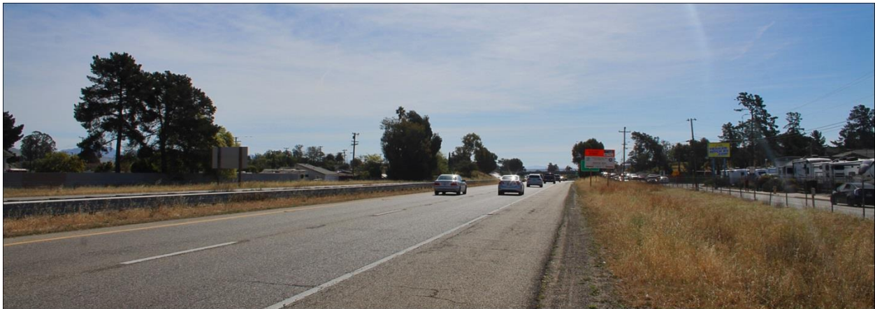
Figure 4.1-12. View along southbound US 101 approaching Tefft Street.
