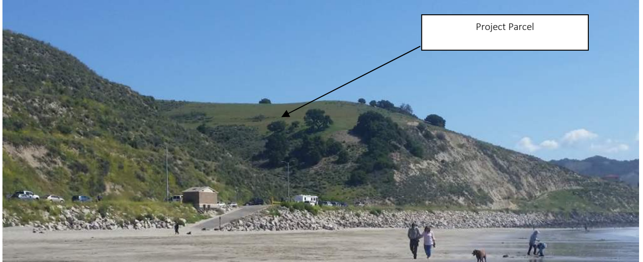
Figure 50: View of Project Location from below Avila Beach Drive, looking east (Photo taken 2016)
