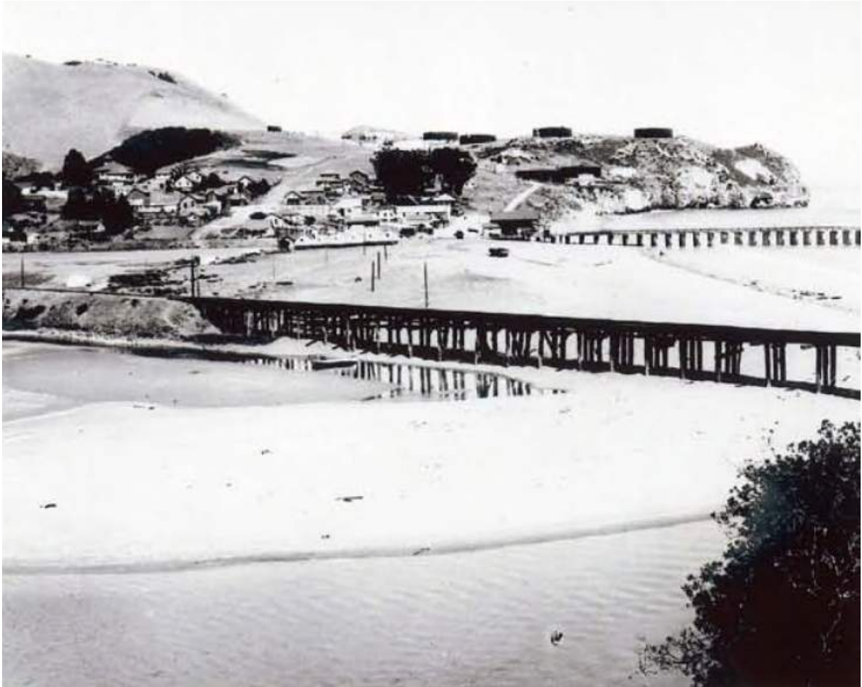
Figure 32: 'San Miguel' Spur Track with Avila Beach and Union Oil Tank Farm in Background (1918) (San Luis Obispo Historical Society)
