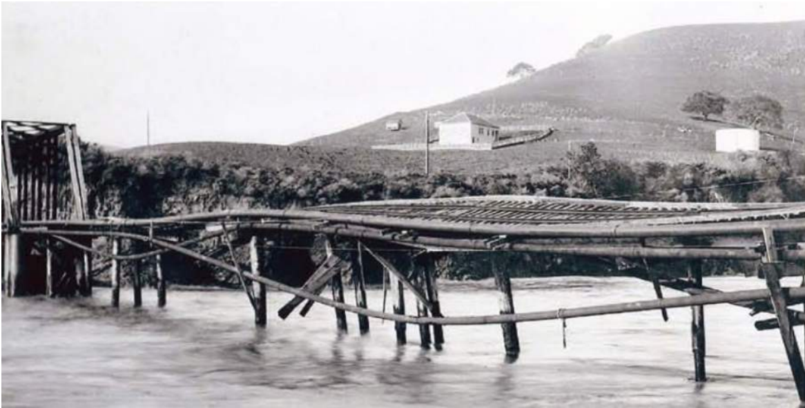
Figure 30: Pacific Coast Railway Bridge over San Luis Creek after storm damage in 1914 (Looking west) (San Luis Obispo Railroad Museum, Unocal Album)
