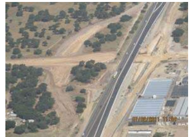
Construction of the Willow Road Project in Nipomo began in 2010.
