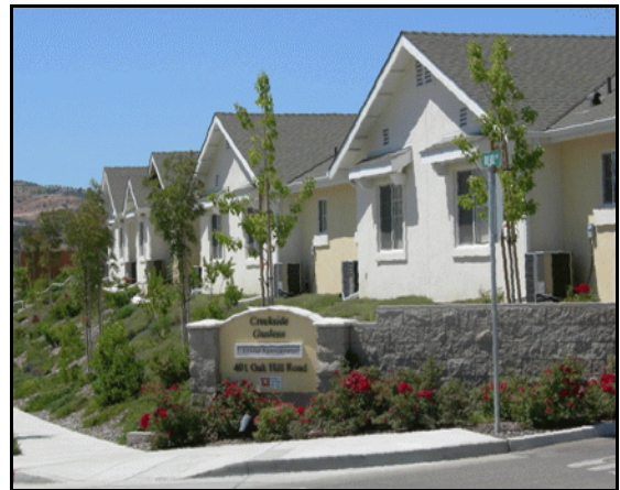
Figure 1-10: Creekside Gardens affordable housing
