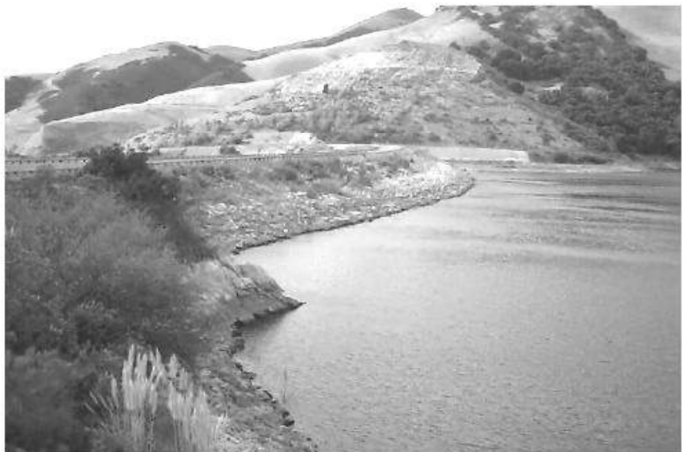
Lopez Dam will be strengthened to reduce its vulnerability to earthquakes.
