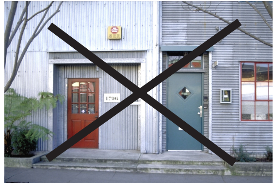
Corrugated Metal (Not Allowed)
