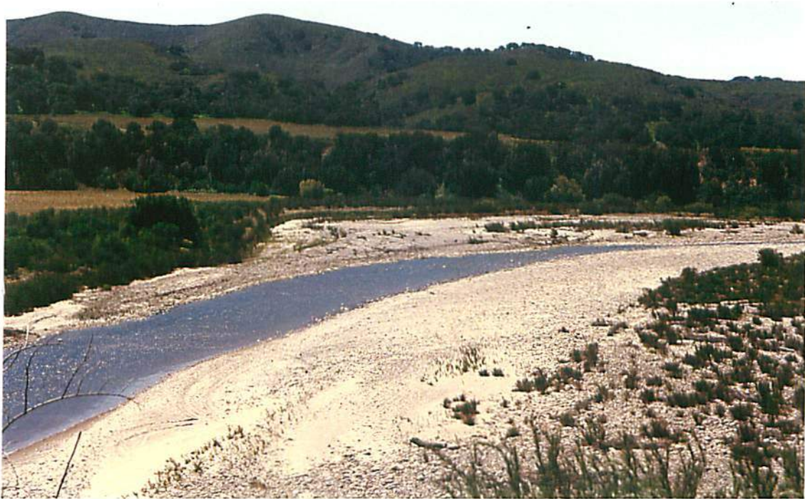
Erosion of Agricultural Lands Along the Sisquoc River
