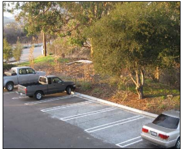
Figure 5.5 Porous Concrete Parking Lot Porous concrete was used in lieu of traditional asphalt to protect the oak tree adjacent to the parking lot. Source: Wallace Group.
