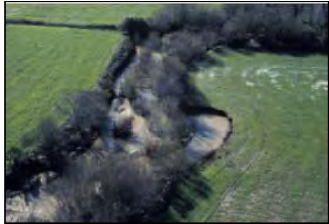
Figure 2-2 Bank scour along San Luis Obispo Creek (Source: USFWS)
