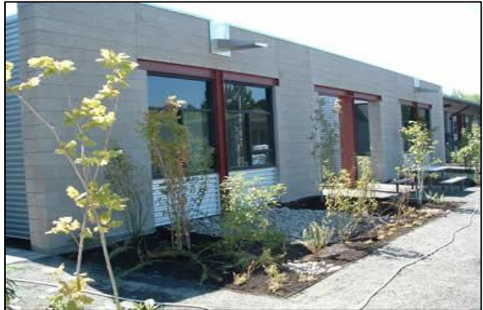
Figure 5.3 Roof scuppers are used to direct runoff through planters. This practice reduces the overall volume of runoff leaving the site during small storms.
