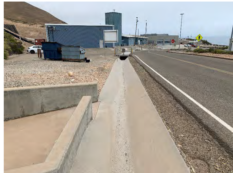
Photo 12: South-facing view of concrete-lined ditch (drainage 28a) within the survey area.
