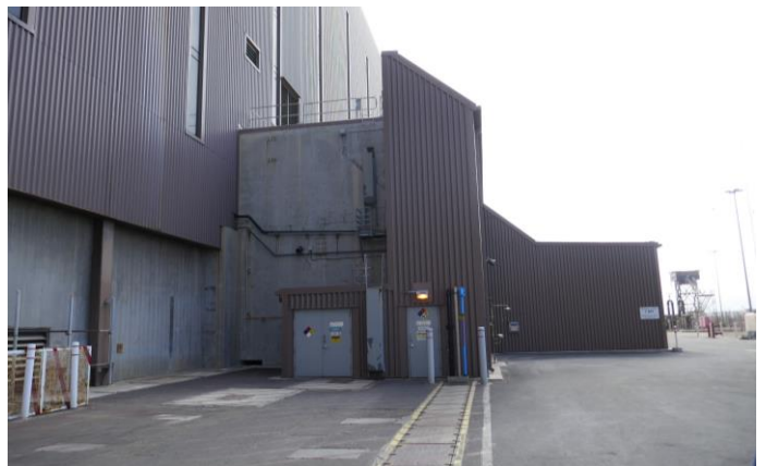
Figure 5: One of two one-story additions at the west façade of the Turbine Building enclosing the structural buttress reinforcements and additional equipment, looking south. Source: Page and Turnbull, 2021.
