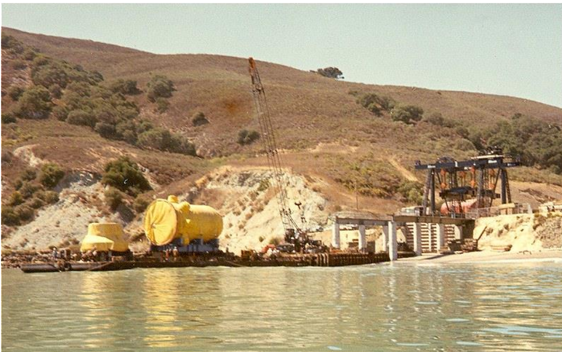
Figure 17. Arrival of the reactor vessel for Unit 1 at the barge landing at Port San Luis in September 1970. Source: Pacific Gas and Electric Company.
