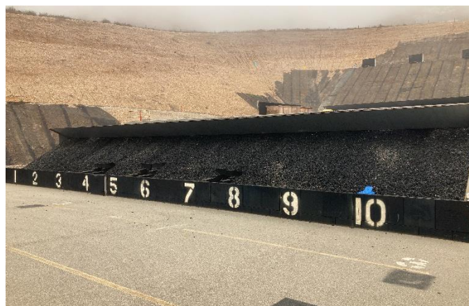
Figure 4: Detailed view of backstop at firing lanes. Source: Page and Turnbull, 2021.
