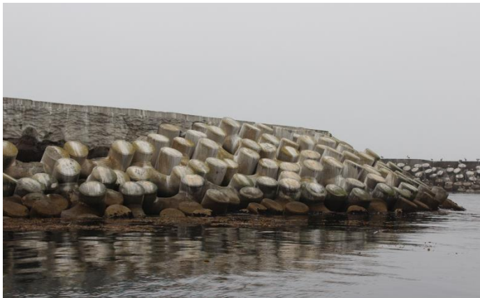
Figure 1: East Breakwater from Intake Cove, with visible concrete tribars, looking west.
