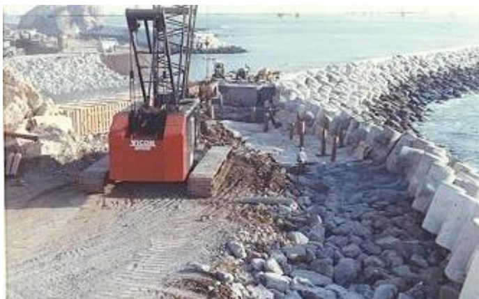
Figure 3: 1971 photo of West Breakwater under construction, looking south. Source: PG&E Archives.
