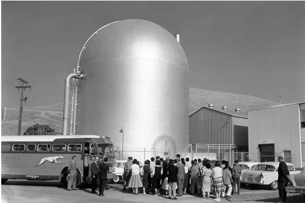
Figure 5. The Vallecitos Nuclear Power Plant (undated). Source: Pacific Gas and Electric Company.
