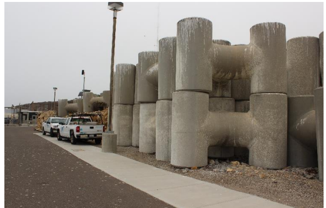
Figure 2: Stored concrete tribar at west side of Intake Cove, looking north.
