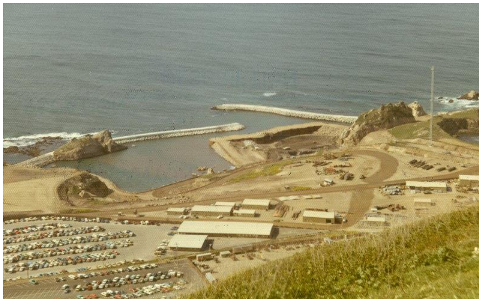
Figure 23. Support buildings and structures in the fabrication yard adjacent to the intake cove, circa late 1971-early 1972, with the triangular-shaped area corresponding to Parking Lot 6 in Zone 5 and the two larger buildings (demolished) in the foreground at present-day Parking Lot 7 in Zone 6. The completed breakwaters and coffer dam for construction of the Intake Structure are visible in the intake cove. Source: Pacific Gas and Electric Company.
