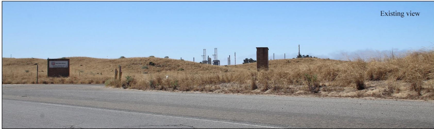
Figure 4.1-6 Existing and Proposed Views from KVA-1 (State Route 1 near the SMR Entrance)
