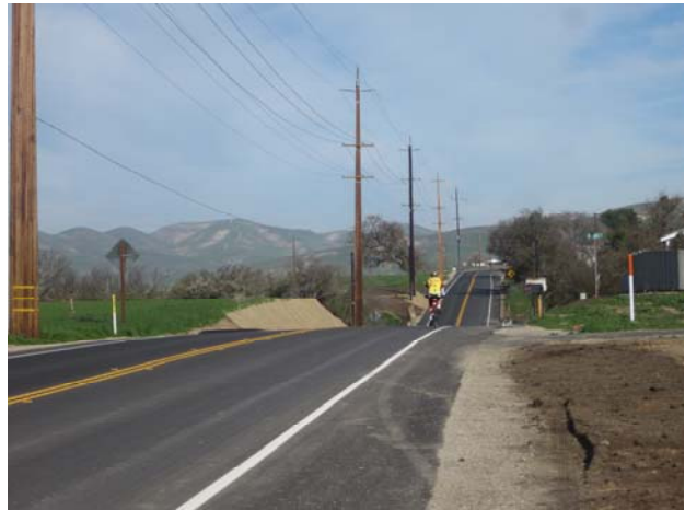
River Road Widening – San Miguel
