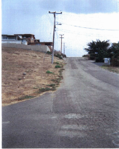
Figure 11: 4-inch on Stuart
