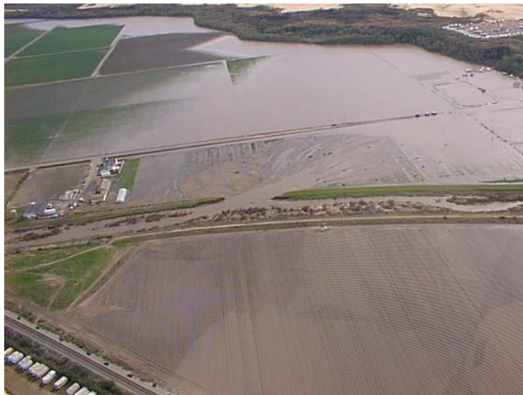
Photo 2. Oblique photo of flooding in the Cienega Valley following the levee breach of March 2001 (looking south).
