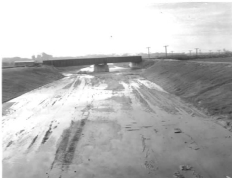
Photo 1. Constructed trapezoidal channel at UPRR bridge in 1958.
