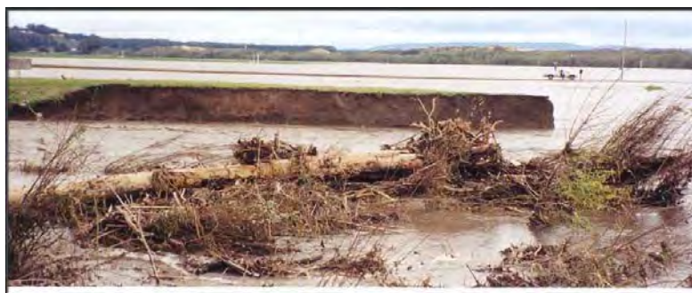
Photo 3. Close-up view of the levee breach and flooding of farmland in March 2001 (looking at south levee from north levee).
