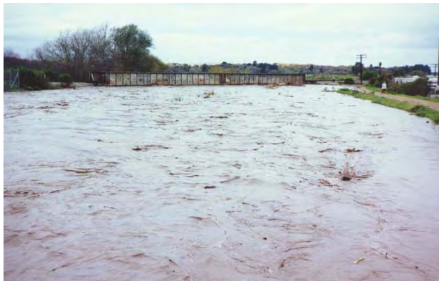
Photo 11. Union Pacific Railroad (UPRR) bridge during the 2001 flood.
