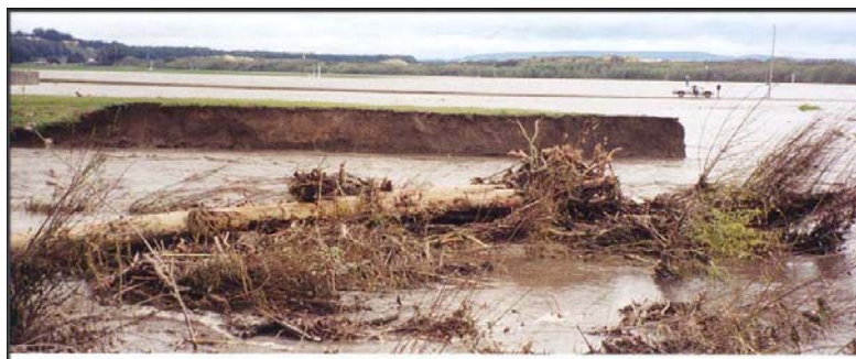
Photo 3. Close-up view of the levee breach and flooding of farmland in March 2001 (looking at south levee from north levee).
