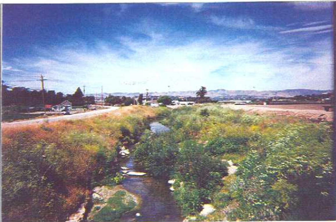
Photo 4: Segment 3. Upstream view of Arroyo Grande Creek flood control channel from Highway 1 crossing. Sediment with riparian/ruderal/channel bank scrub along right side to center of photo is proposed for removal from work area 11. Steelhead observed along boulders in center of photo.
