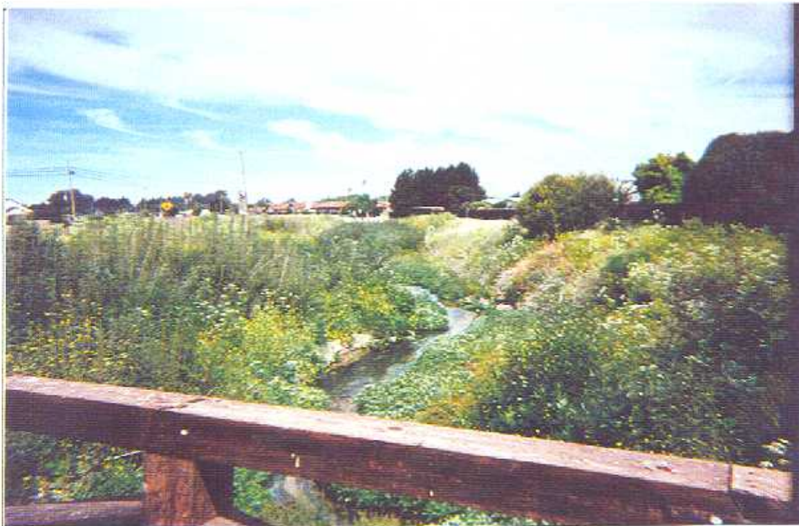
Photo 2: Segment 1. Downstream view of Los Berros Creek overflow channel from Century Lane bridge crossing. Sediment with riparian/ruderal scrub on both sides of the upper bank of levee are proposed to be removed from work areas 2 left and 3 left.
