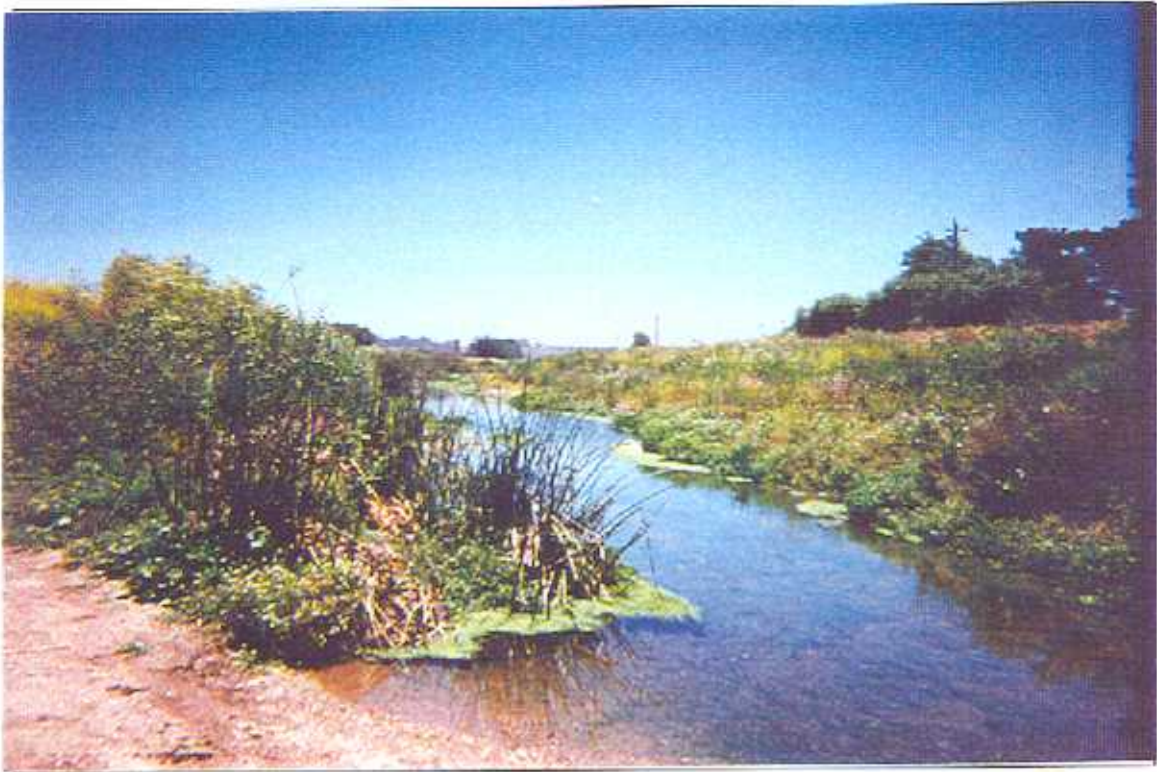
Photo 11: Segment 7. Upstream view of Arroyo Grande Creek flood control channel from access road crossing #5. Sediment with riparian/ruderal scrub on left bank is proposed for removal from work area #28.
