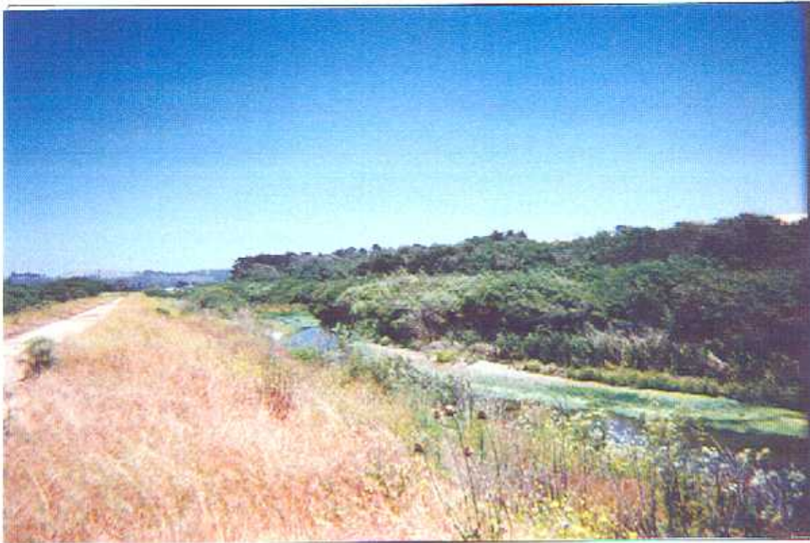
Photo 13: Segment 8. Upstream view of Arroyo Grande Creek flood control channel from north bank of levee. Sediment with ruderal scrub patch on left bank, on center of photo is proposed for removal from work area #32.
