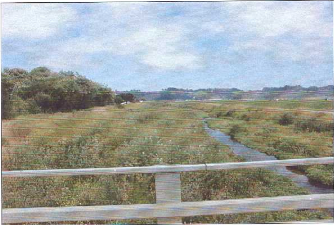
Photo 7 Segment 5. Upstream view of Arroyo Grande Creek flood control channel from 22 nd Avenue Bridge. Sediment with riparian/ruderal scrub along left bank in photo is proposed for removal from work area #18.
