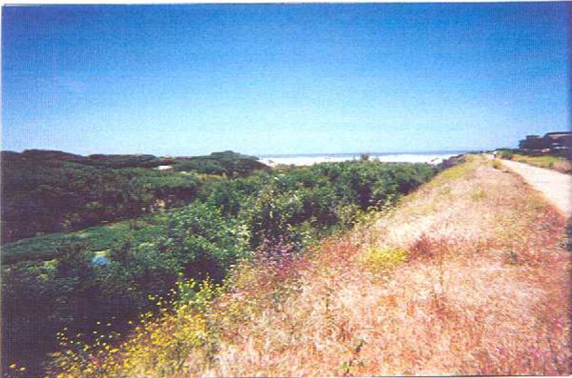
Photo 14: Segment 8. Downstream view of Arroyo Grande Creek flood control channel from north levee bank. This area is not proposed to be removed.
