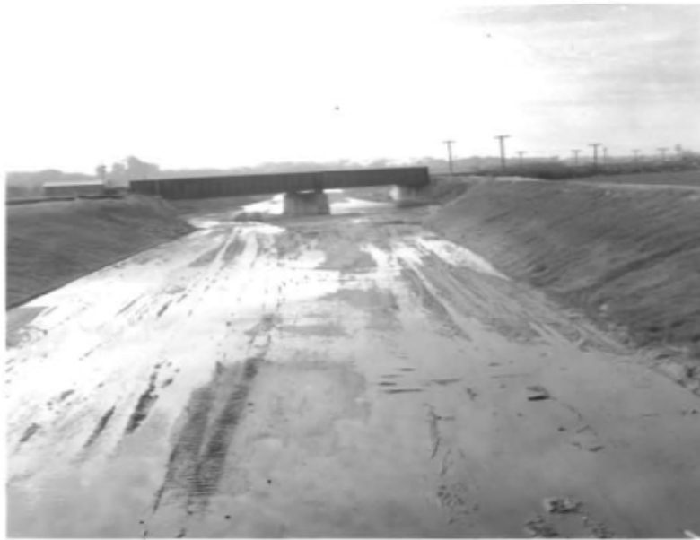
Photo 1. Constructed trapezoidal channel at UPRR bridge in 1958.
