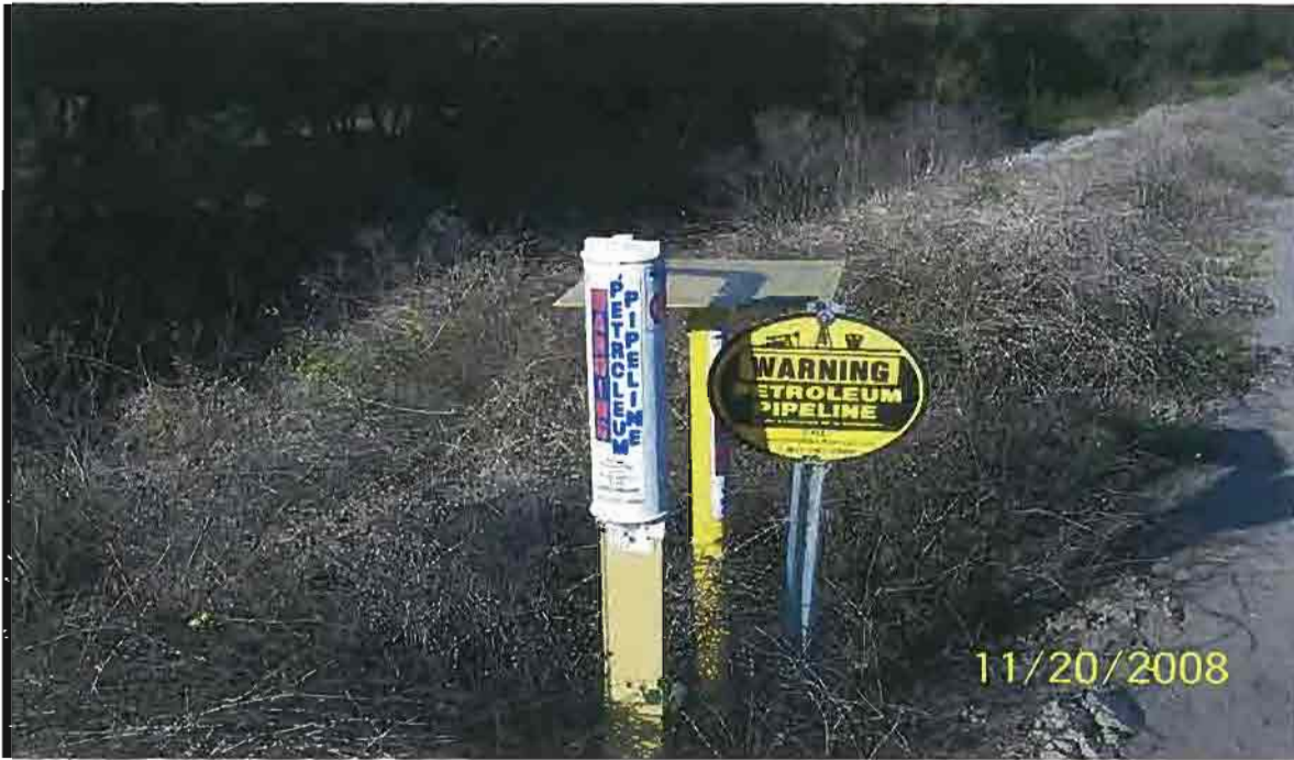
View of a petroleum pipeline marker located along the creek bank parallel to Halcyon Rd.
