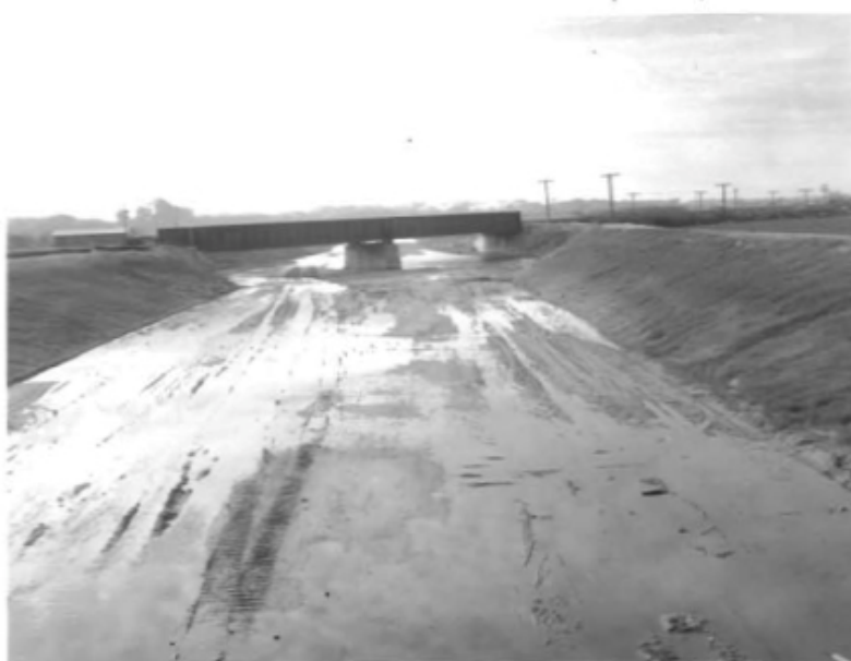
Photo 1. Constructed trapezoidal channel at UPRR bridge in 1958.
