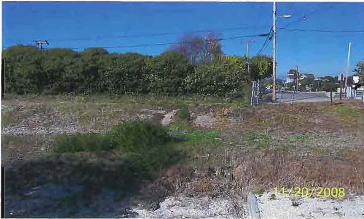
View of the creek bottom looking north at the site located at the intersection of Valley Rd. & Los Berros Rd.
