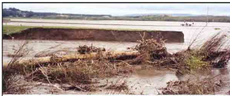
Photo 3. Close-up view of the levee breach and flooding of farmland in March 2001 (looking at south levee from north levee).
