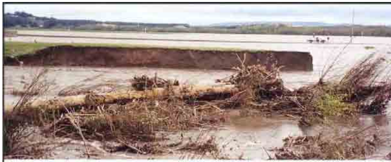
Photo 3. Close-up view of the levee breach and flooding of farmland in March 2001 (looking at south levee from north levee).
